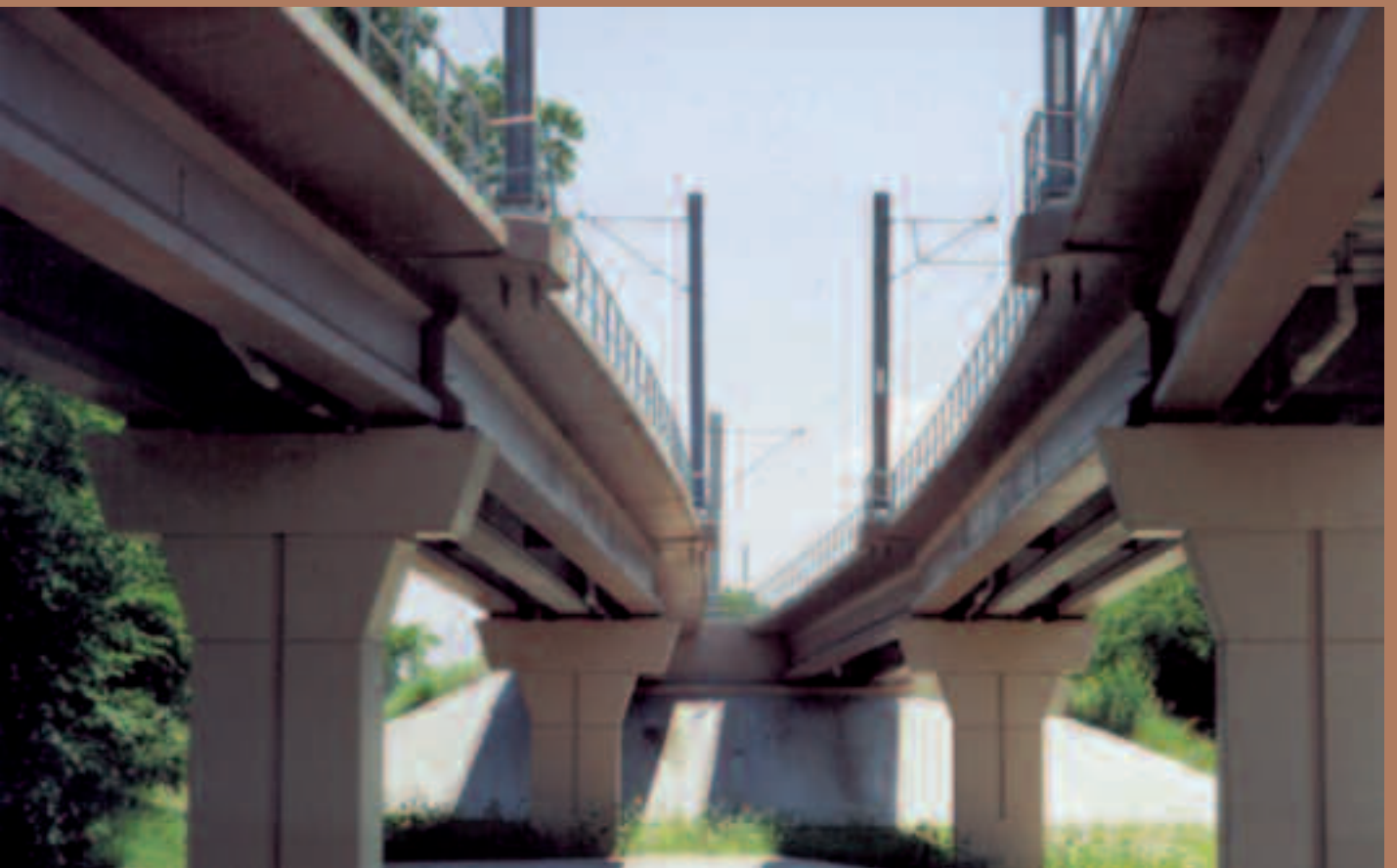
NC-3 light rail - structure - TX
