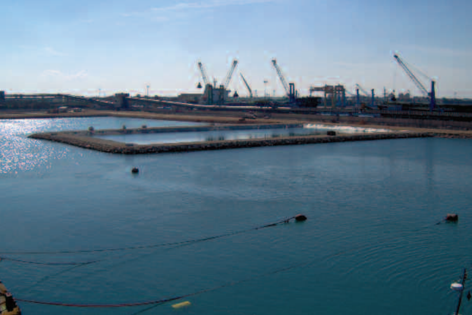
Banchina Costa Morena, Brindisi • Costa Morena wharf at Brindisi harbour
