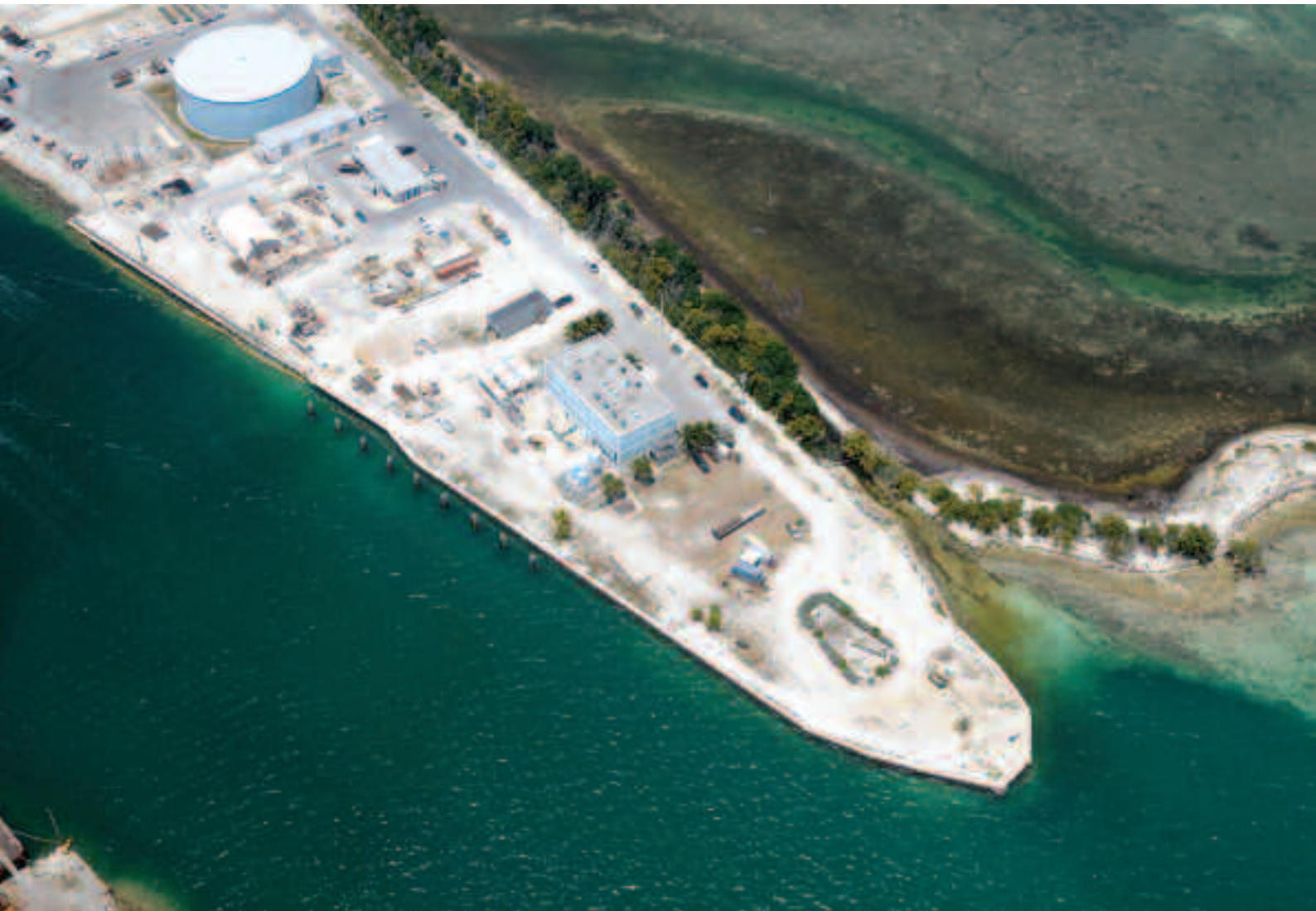
Stock Island Bulkhead Replacement Key West - FL
