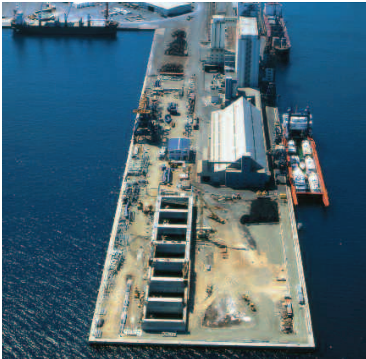
Banchina Boselli, Porto di Savona • Savona Port, Boselli quay and deposit for bulk terminal
