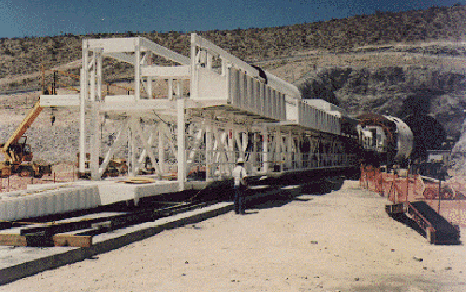
Umiray-Angat Tunnel - Philippines
