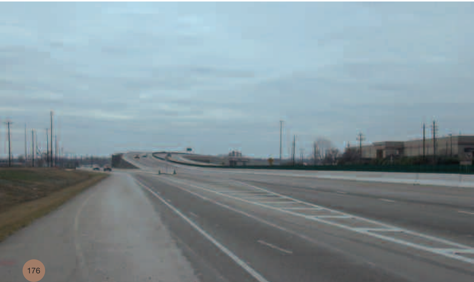
Austin 183 overpass - TX
