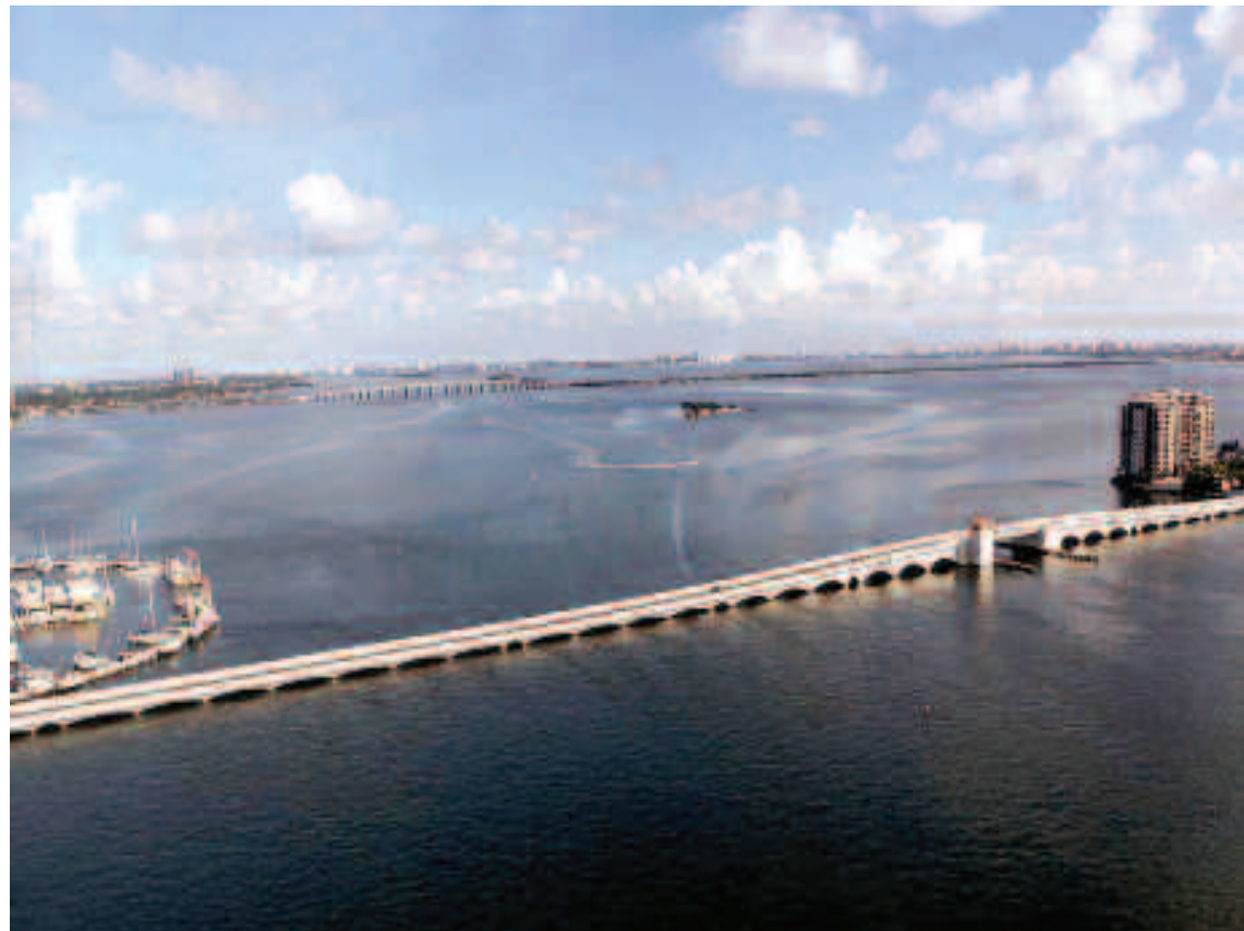
Venetian Causeway Bridge Historical Reconstruction / Renovation Project - Miami Beach - FL
