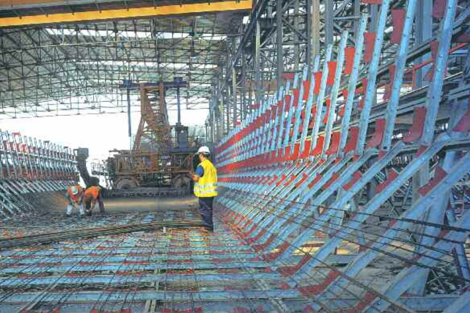
Armatura viadotto ferroviario • Reinforced concrete steel cages for a rail flyover
