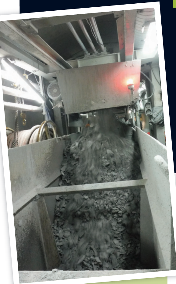
Top: Hexagonal segments are cast at the on-site segment factory using Fama moulds Above: The moving tripper conveyor efficiently loads the muck wagons
