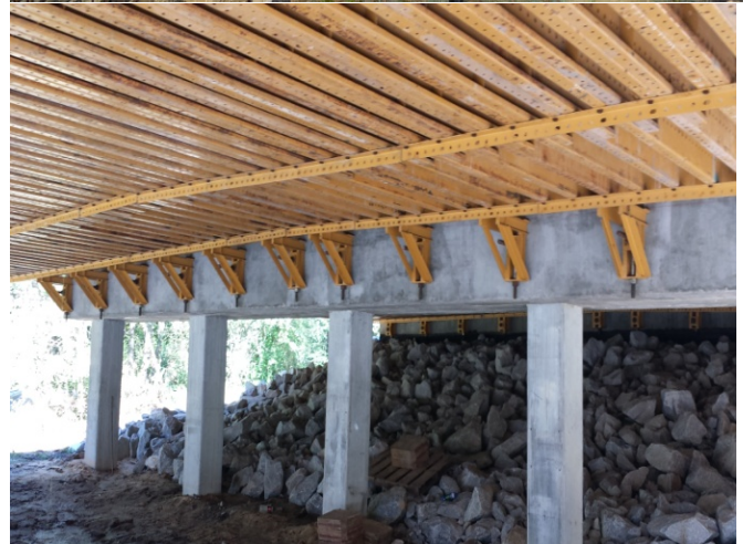
EFCO Flat Slab Form System (Span 6)
