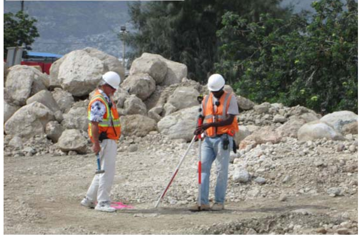
Setting up RO-RO Test Piles
